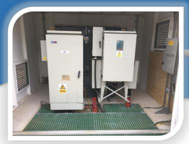
1500 kva Package Substation within the GRP Housing
