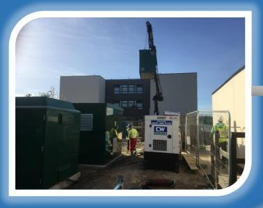
1500 Kva Substation LV Customer Switch room and bespoke Gas Kiosk.
